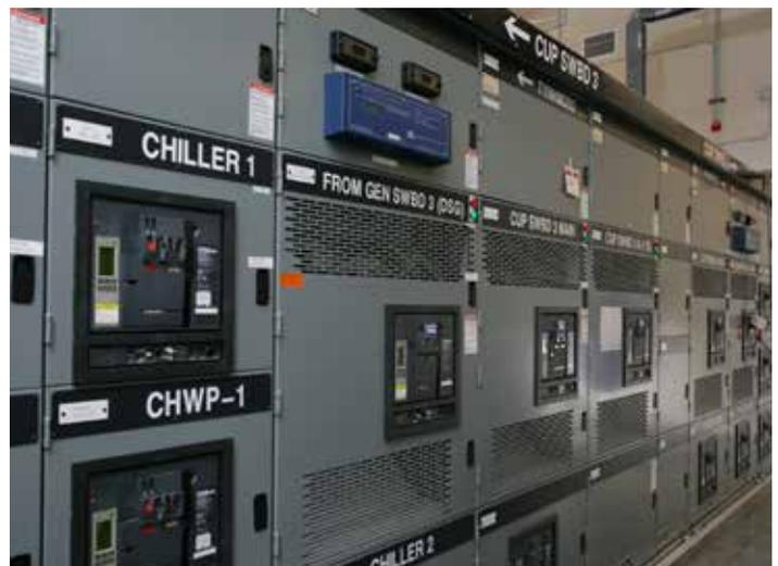
Drawout switchgear is often needed in healthcare facilities to meet code requirements for selective coordination.
