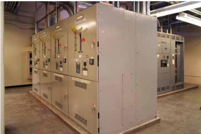
Automatic transfer switches are a critical item of electrical systems that require arc flash-rated personal protective equipment, or PPE, during annual inspections.
